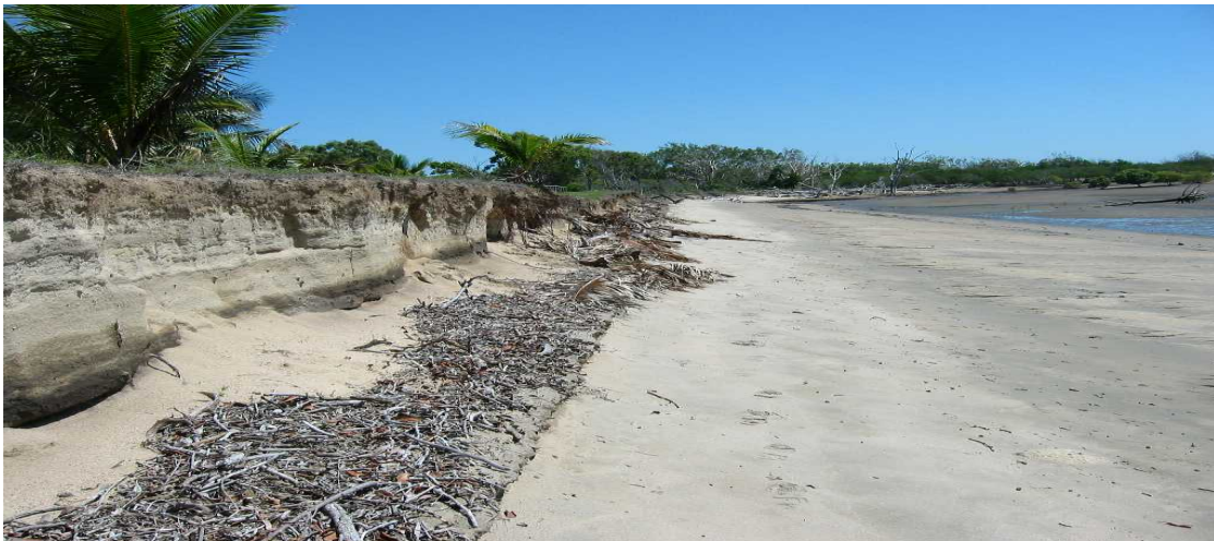
Figure 1: McEwens Beach erosion scarp
