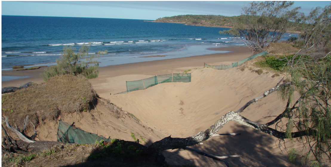
Figure 5. Sand blow area.
